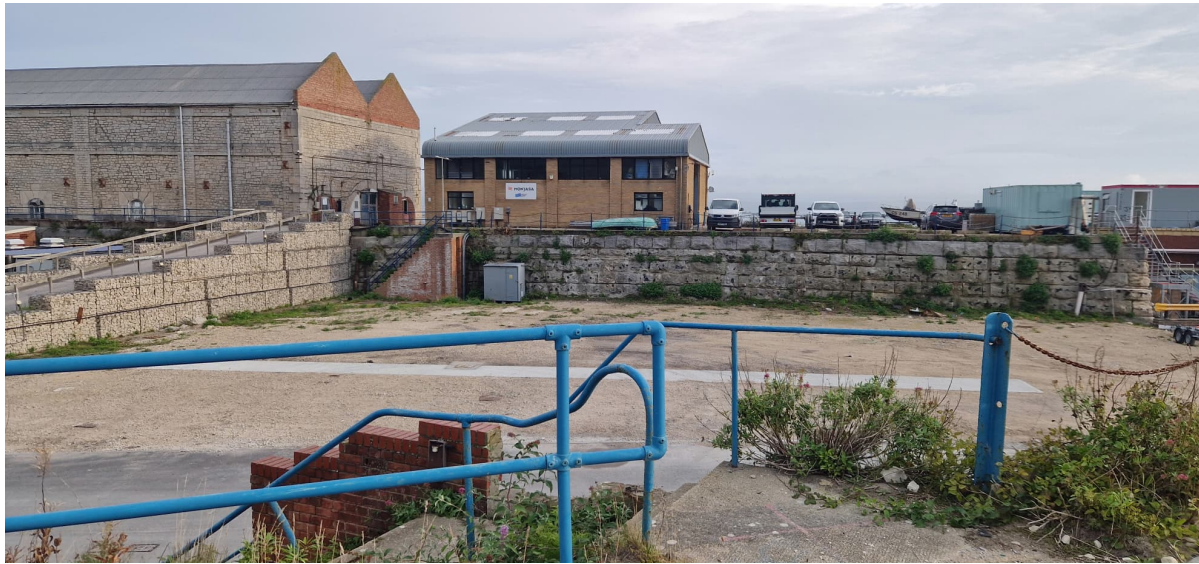
Figure 2– PBUK control room, lube oil store, and workshop
