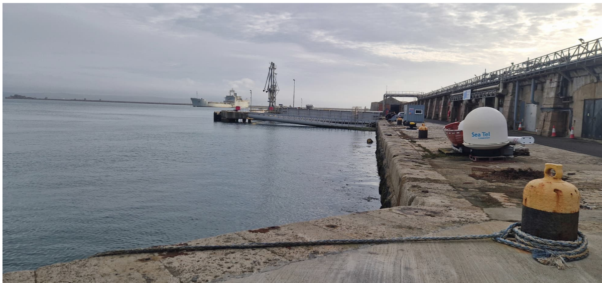
Figure 4 – PBUK fuel bunkering berth
